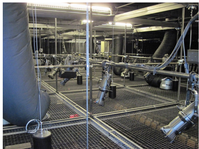
Figure 7 Tension Wire Grid
